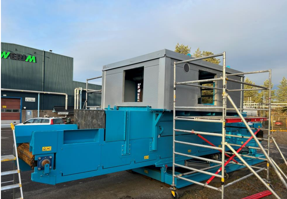
Analysis station for heavy scrap - ongoing mounting of parts
